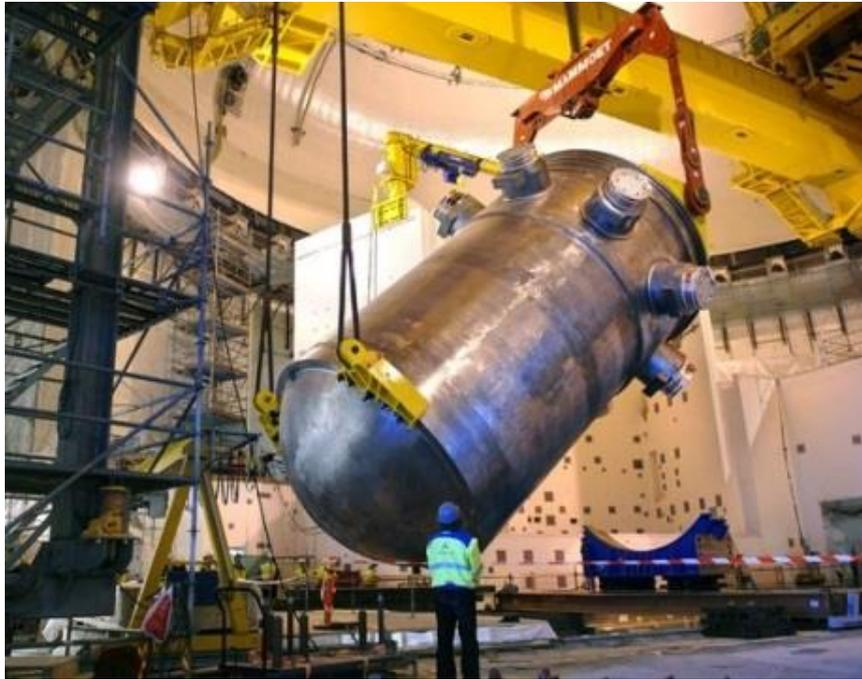
*EPR Reactor pressure vessel in the installation process at Oikiluoto (June 2010 – image: Framatome).*
